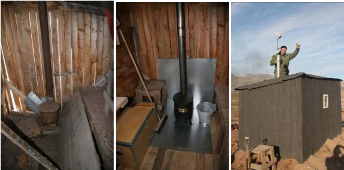
Left and middle: Interior of Norma hytta [411-2] before and after renovation. Right: Anders Ibsen putting on roofing felt.
