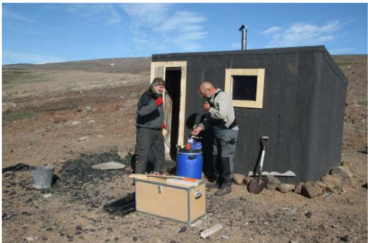
Mellemhuset [367-2] during renovation. From left Torben Krogh Johansen and Per Ibsen.
