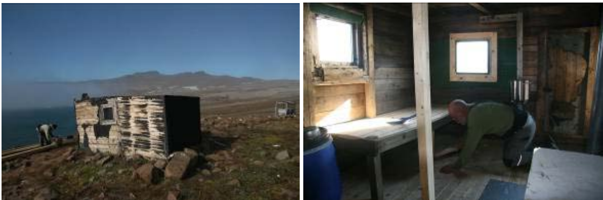
Dahl Skær hytten [412] before and during renovation. A new floor was put on the existing floor in the hut.
